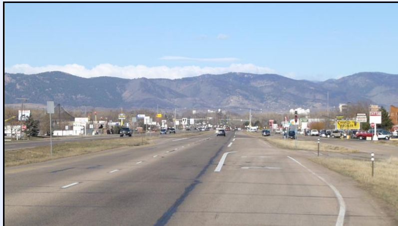
CLP/NPB Eastern terminus (looking west) showing the byway's commercial/industrial character east of Fort Collins.
